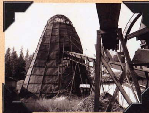
TEPEE BURNER Get rid of all those lumber scraps, bark, trimmings and sawdust! Use our tepee burner to burn your wood waste.
