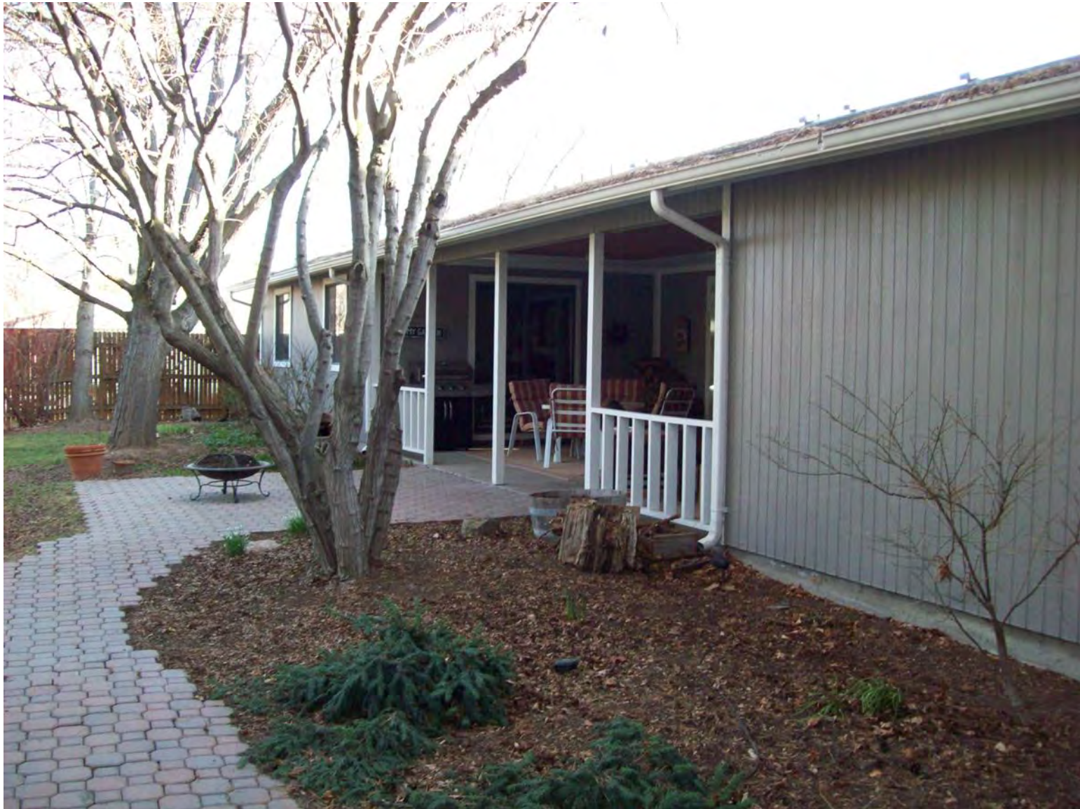
Existing Patio, Prior to Remodel
